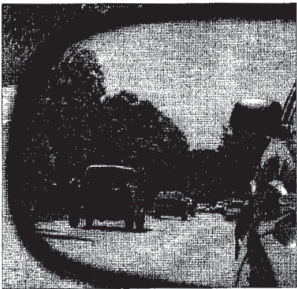
Thanks to a little roadwork conducted by the entrance of Pea Ridge National Military Park, traffic was backed up on a two-lane portion of U.S. Highway 62 on Wednesday morning. As the Arkansas Highway and Transportation Department continues its road-widening project toward Garfield, this may become a familiar site.
